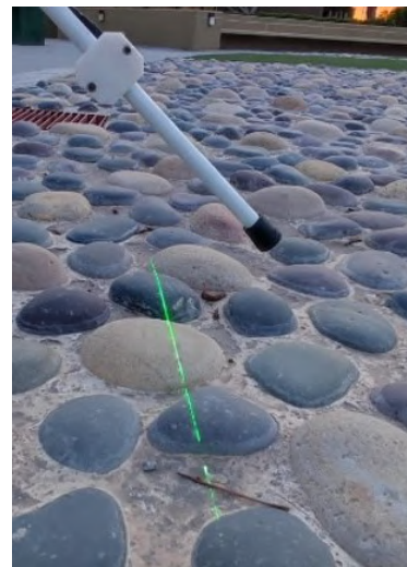
Fig. 14. Fourth Stage. Uneven Surface
