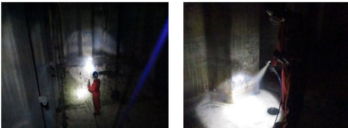
Figure 5-17: VCI fogging fluid to treat void spaces and tanks
