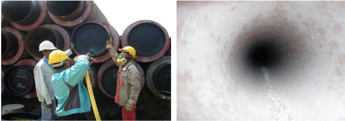
Figure 5-22: Preservation of steel pipes with VCI fogging powder
