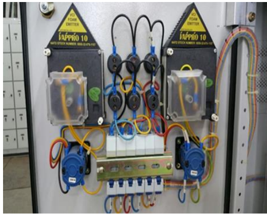
Figure 5-10: VCI emitters and pouches used in large control panels, electrical power supplies
