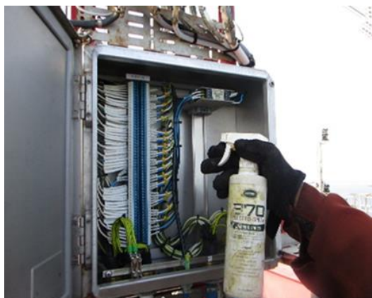
Figure 5-11: Application of VCI electronic spray to electric circuits and relays
