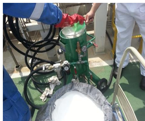
Figure 5-12: VCI powder is fogged to preserve the piping system
