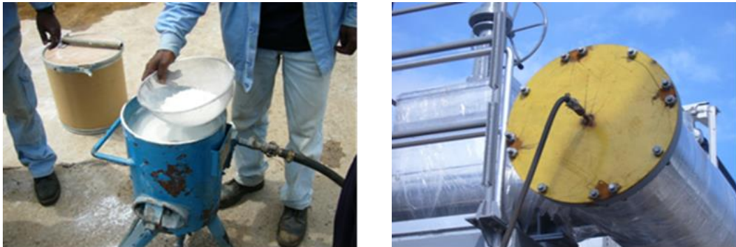
Figure 4-19: Used VCI powder to fog piping system
