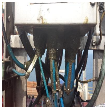
Figure 5-15: VCI wrapping tape to protect flanges and valves
