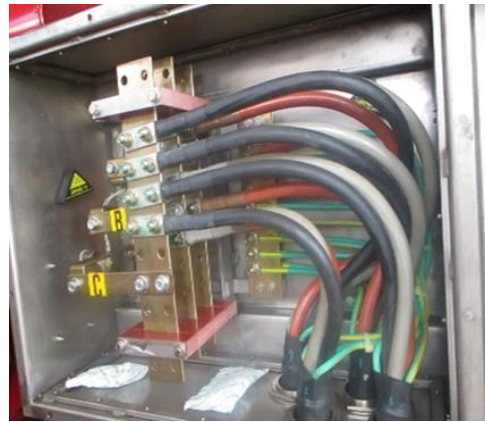
Figure 5-10: VCI emitters and pouches used in large control panels, electrical power supplies
