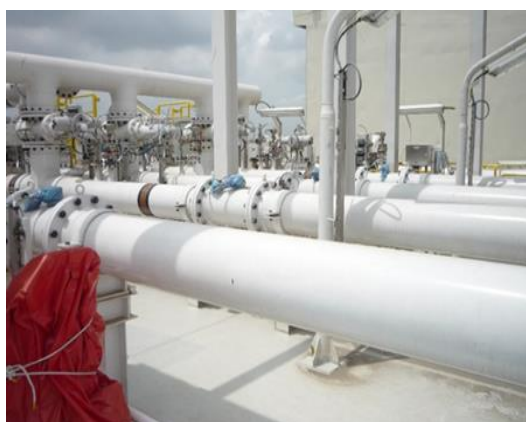
Figure 5-12: VCI powder is fogged to preserve the piping system
