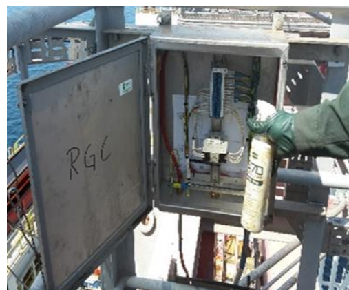
Figure 5-11: Application of VCI electronic spray to electric circuits and relays
