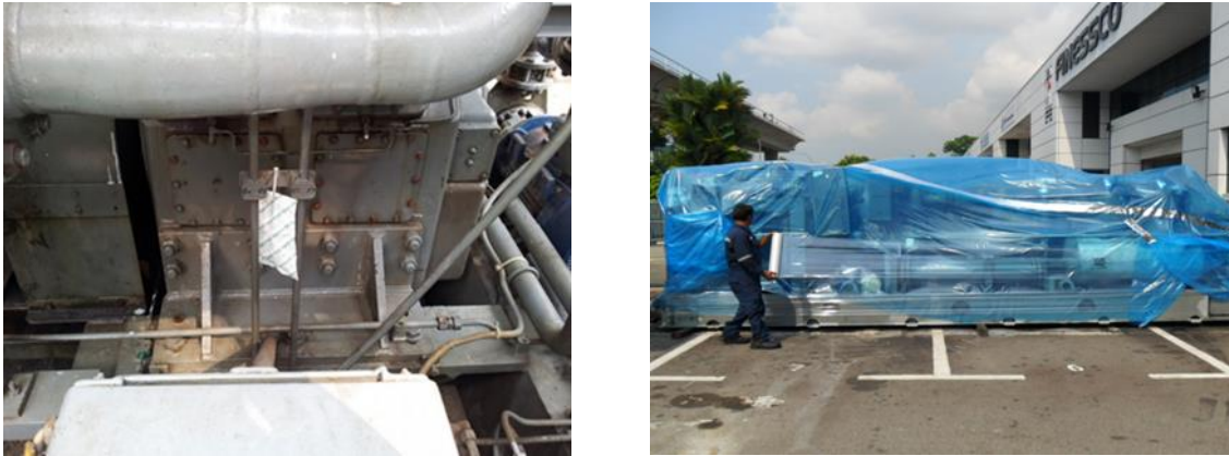
Figure 5-20: VCI pouches to the compressor and wrapped with VCI film
