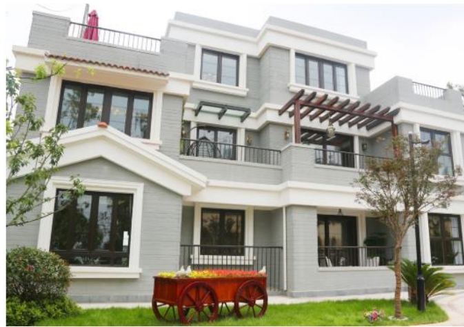
Figura 10. Casa impresa por WINSUN (Fuente: Demonstrating the Viability of 3D Printing at Construction Scale)
