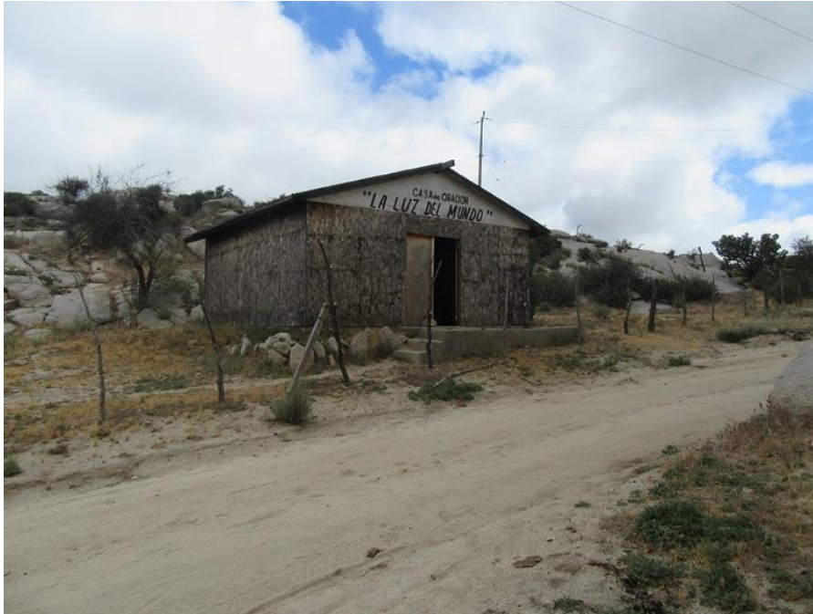
Figure 20. Abandoned church Casa de Oración La Luz del Mundo, converted into Tirsia Flores Castro's workshop and store in 2016. May 7, 2017.
