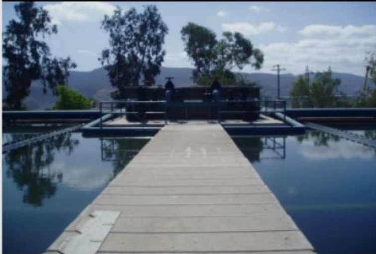
A plant for water treatment and clarification.
