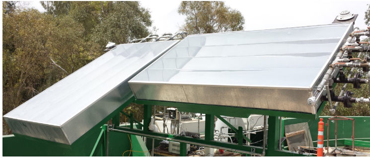
Fig. 4. CPC modules installed in Mexicali, Mexico.
