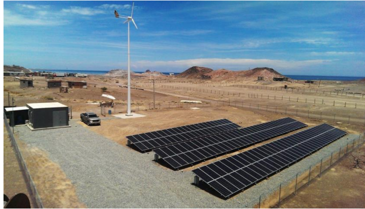
Fig. 1. Microgrid in Puertecitos
