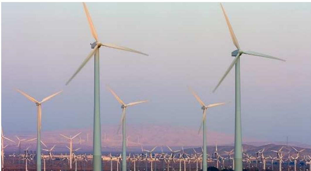
Figura 1.1: Alta Wind Energy Center (AWEC) 1 .
