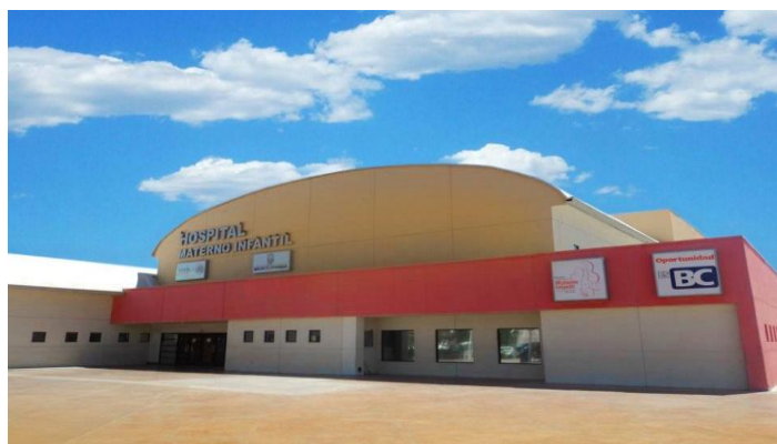
Figura 1. Facha principal del Hospital Materno Infantil, Mexicali, Baja California.
