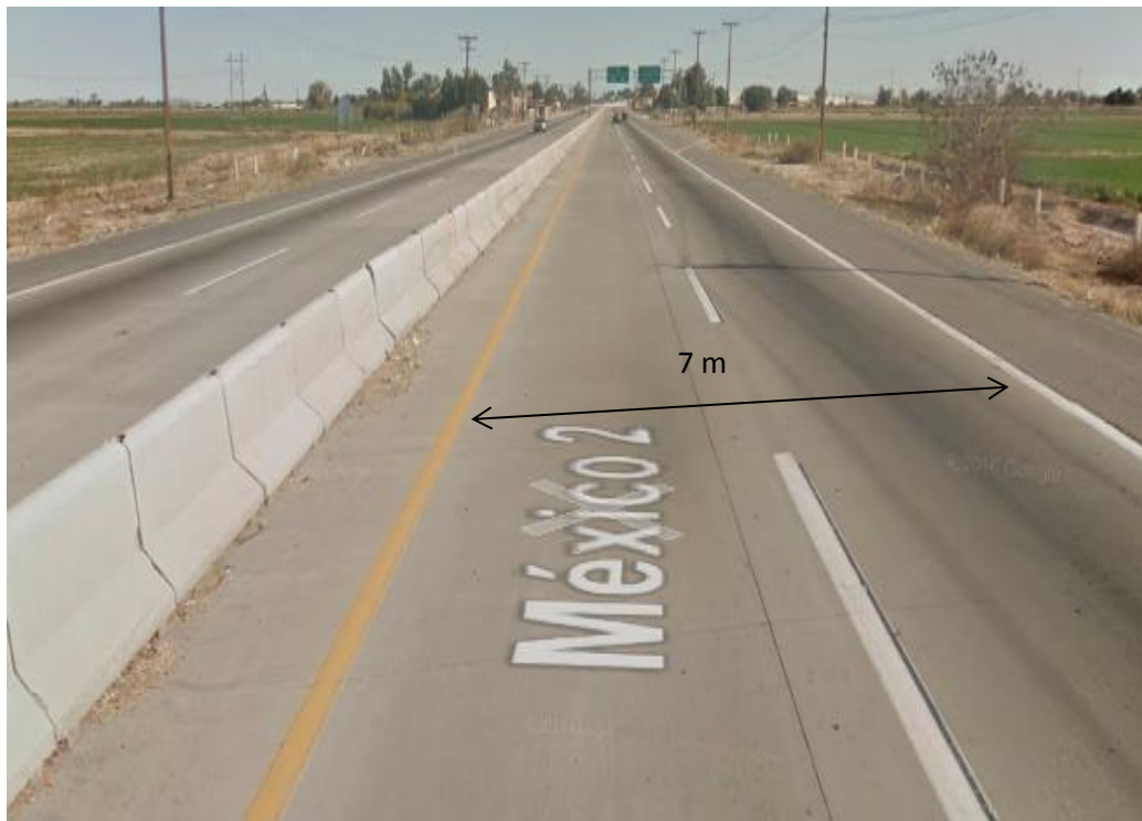
Figura 2-35 Carretera federal primaria 2, Tramo Mexicali-Sonoyta
