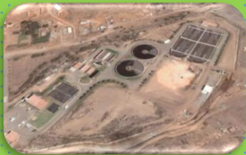
Figura 1. PTAR "El Naranja"
