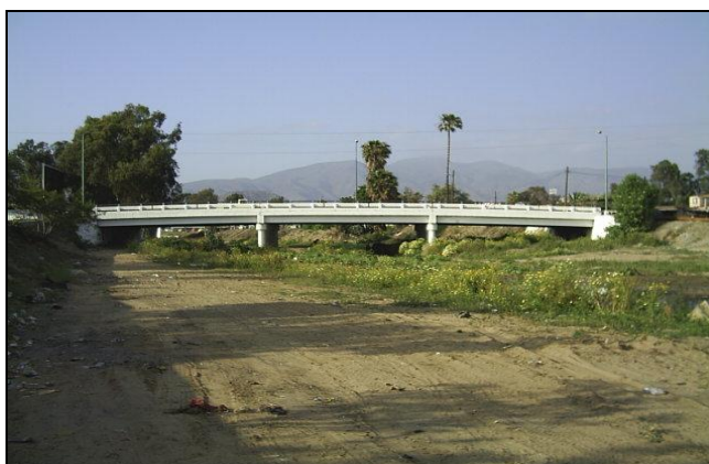
Figure 1 One of the 29 Ensenada urban bridges: Calle 9.
