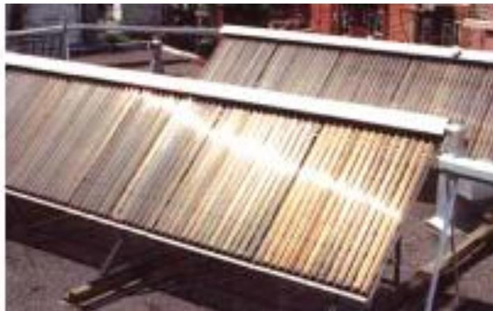
Figura 2.11: Colector de tubos evacuados
