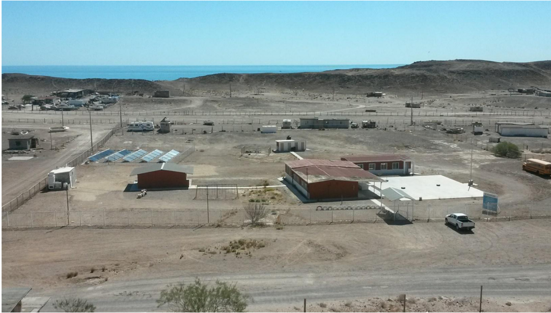
Fig. 3. Puertecitos elementary school and kindergarten, with the absorption cooling system activated with solar thermal energy.
