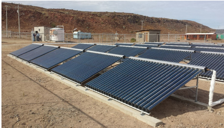
Fig. 2. Thermosolar absorption cooling system of 35 kW capacity installed in the primary school of Puertecitos, Mexico.
